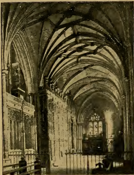
FIG. 76.—SOUTH AISLE OF WINCHESTER CATHEDRAL, ENGLAND.
